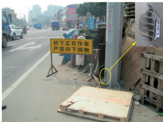
Figure 1. Tyre marks of the front wheel of the motorcycle on the pillar (the next day).
